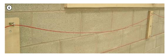
**7a.** Unscrew the eyehook from the Hexagon shaped Thimble and re-fit the eyehook by 3 turns of the thimble to ensure that the eyehook is secure. Leave the maximum thread possible for later adjustment of the rope tension.
