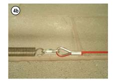
5. For systems over 50m. two Tensioner/Gripper assemblies are provided to enable the maximum tension range to be achieved over longer lengths (there is no Quick Link provided). In this case instead of a QL, fit a Tensioner/Gripper to both ends of the system (See 7a and 7b).
