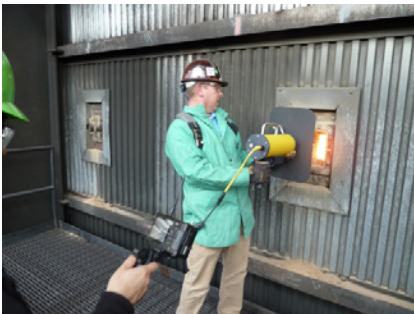
Application of the BoilerSpection-IM
